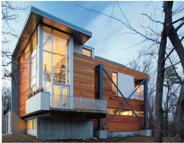
A dramatic glass and aluminum corner and the rich warm tones of natural wood siding on this Massachusetts home belie its considerable salvage content (300 tons of recycled steel beams and concrete from Boston's Big Dig infrastructure project). Credit: Single Speed Design
